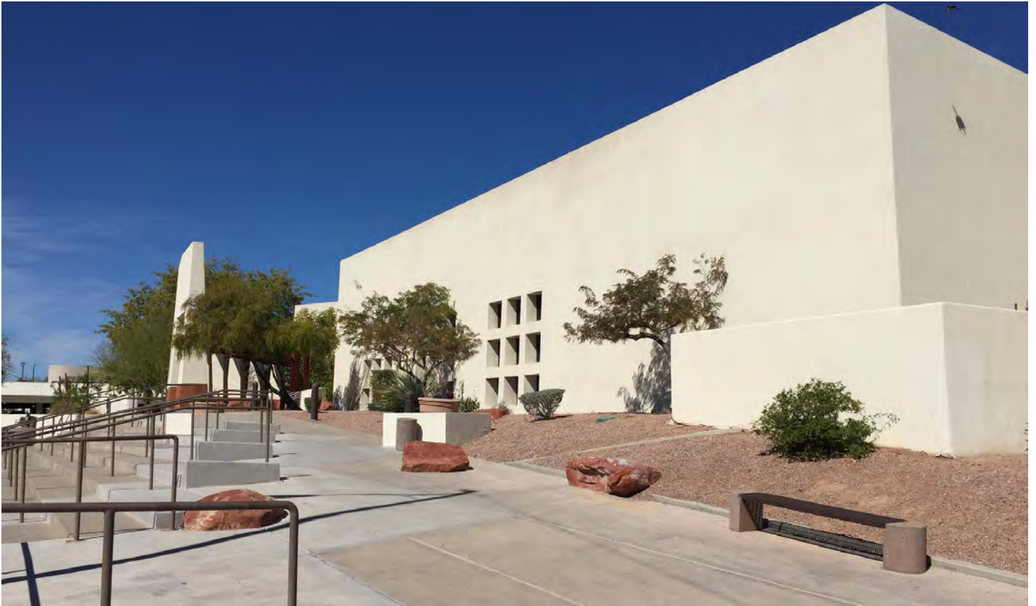
Looking North West
