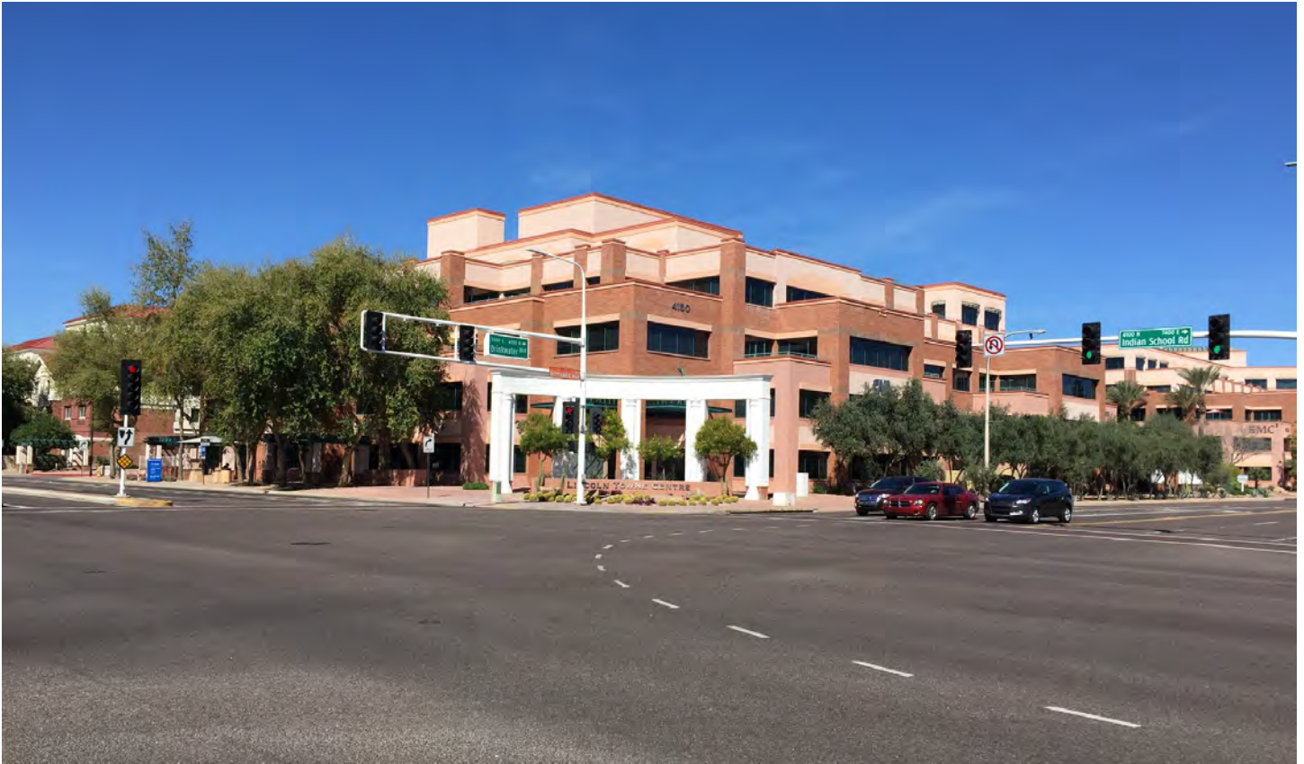
Looking North West
