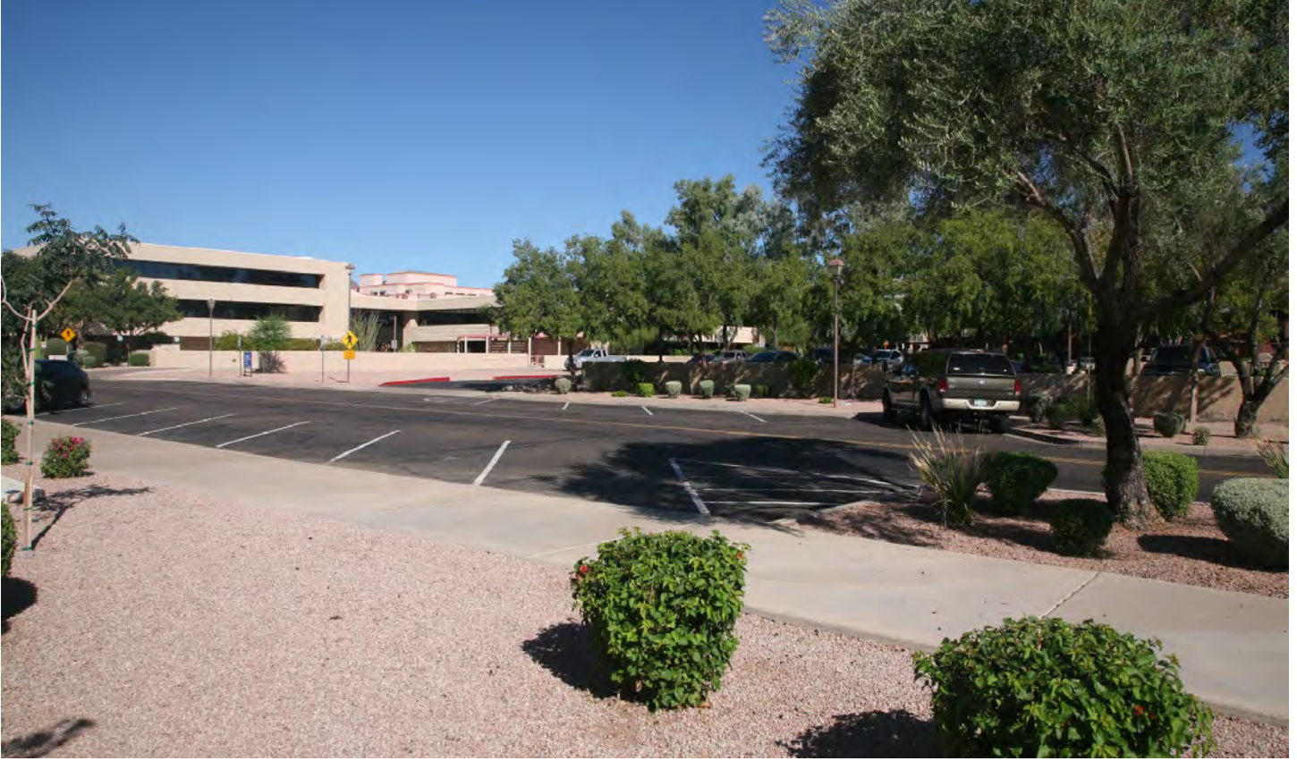
Looking North West
