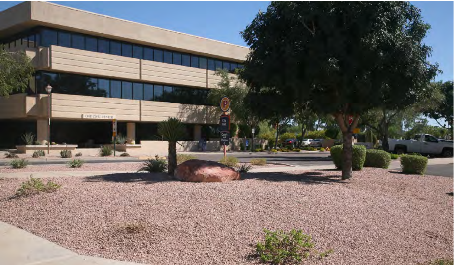
Looking North East
