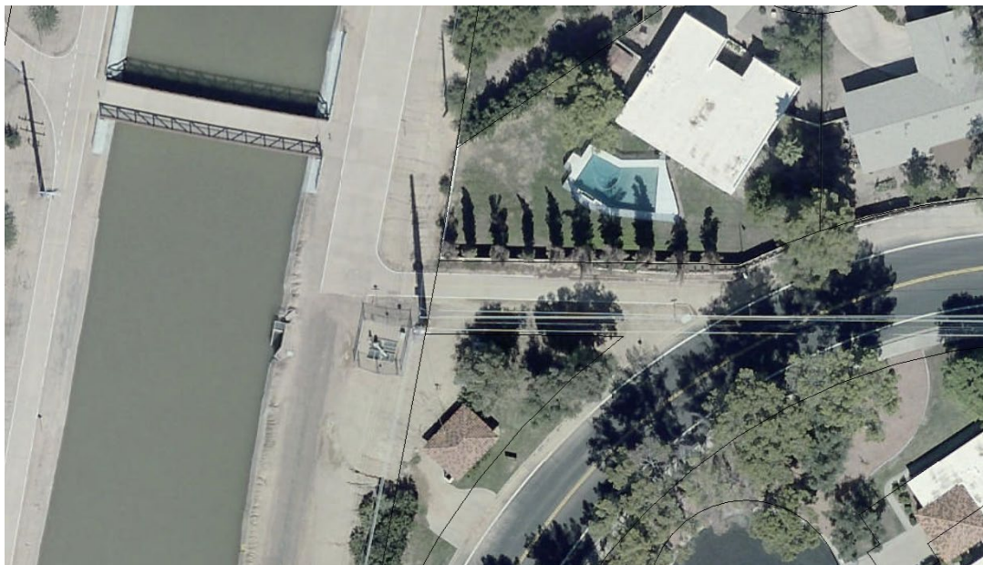
Figure 2 – Arizona Canal Bridge and Path Connection
