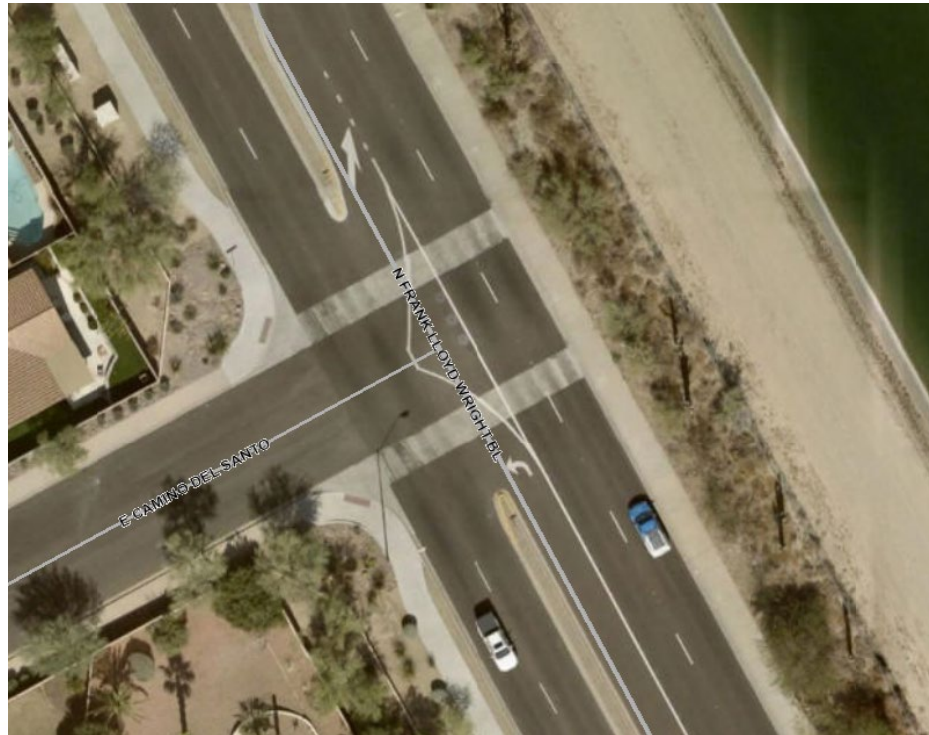
Aerial view of Frank Lloyd Wright & Camino del Santo: LILO Site (painted median)
