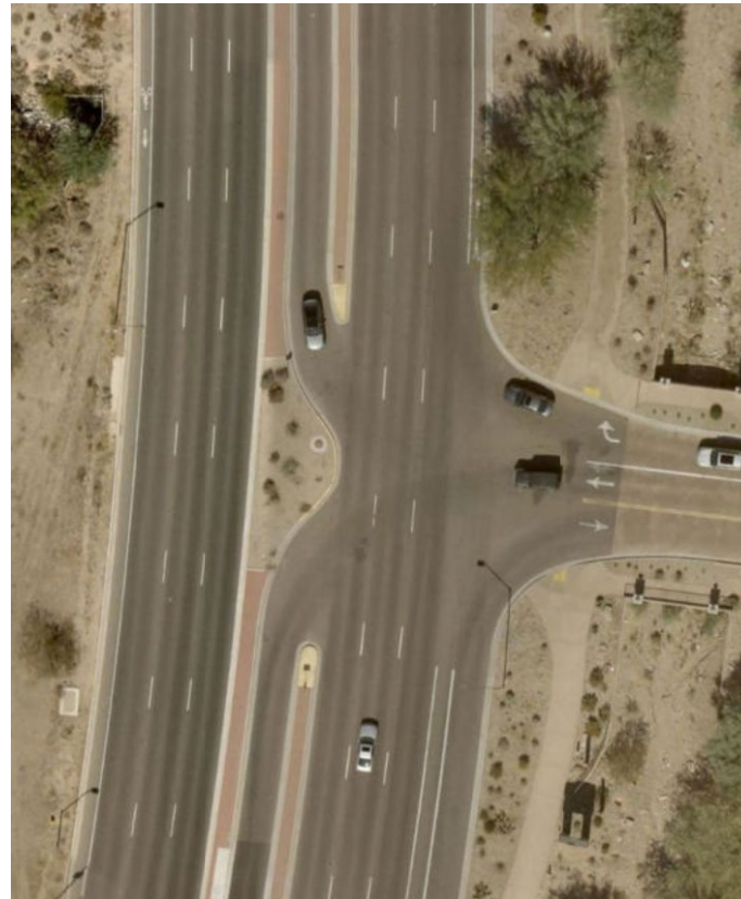
Aerial view of Pima Rd & DC Marketplace: LILO Site (raised median)
