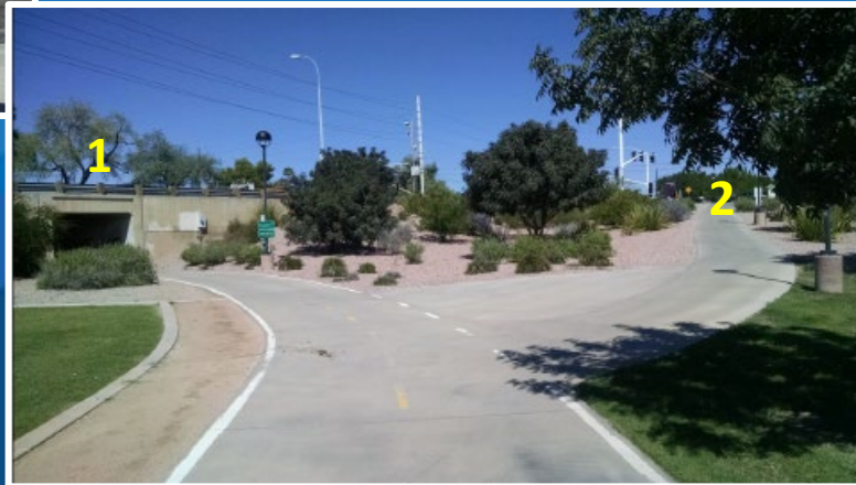
South of the project area, looking NW Existing east/west tunnel (1) and proposed underpass (2)
