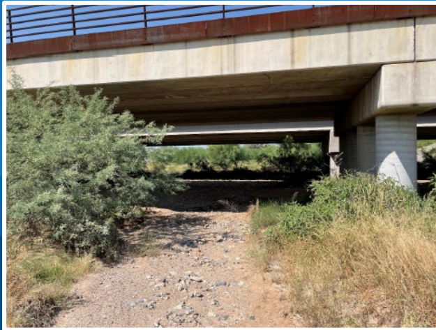
Looking north underneath Existing Bell Road Bridge
