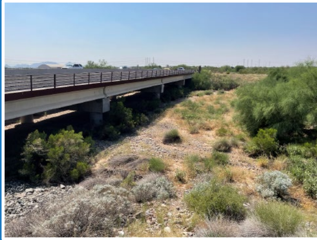
Looking west, on north side of Bell Road Bridge
