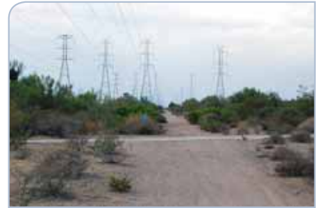
The power line corridor on the northeastern boundary of the Greater Airpark provides electric service to Scottsdale.
