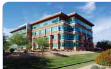
Employment Land Use Area design should consider contemporary expressions of corporate identity.
