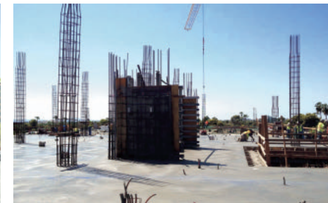
Figure 4: Optima Sonoran Village construction.
