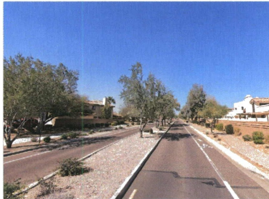
Minor Collector 96 th Street - After
