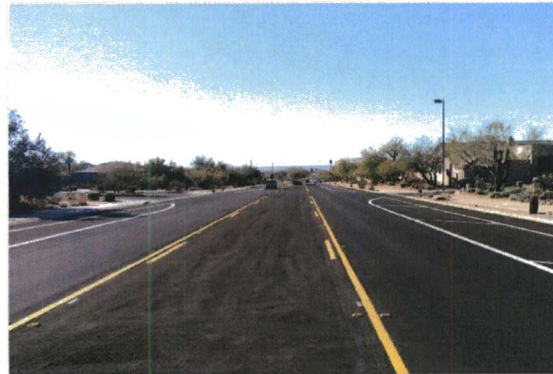
Minor Collector 124 th Street - After
