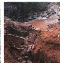
Repair erosion and sedimentation
