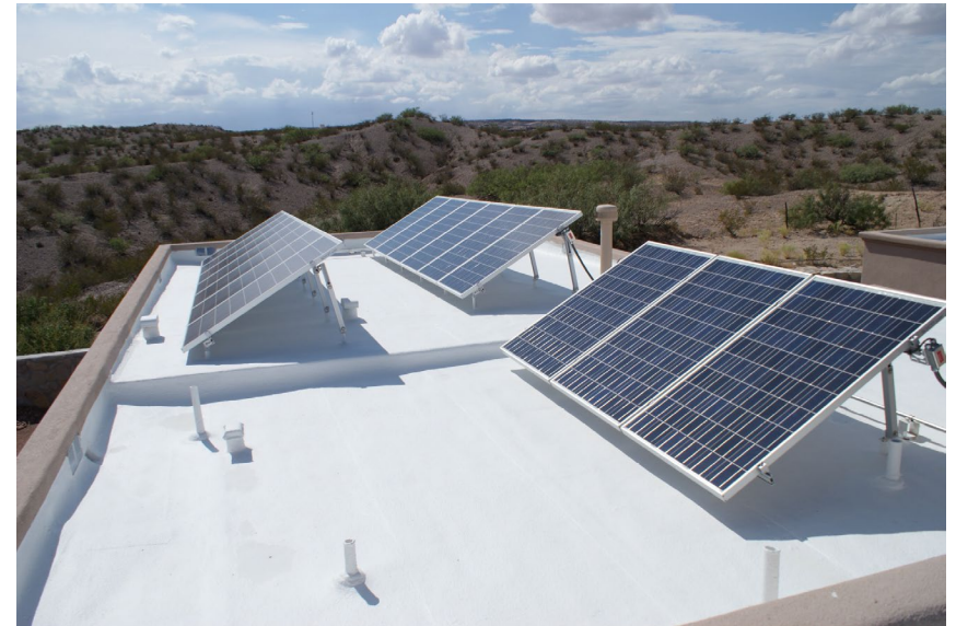
Credit: Carlisle Roof Foam
